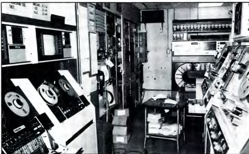
KTHI-TV's tape room houses the station's 1-inch, 2-inch cartridge and cassette tape recording equipment. Machines in this room can be accessed by the master control room or the production control room.
