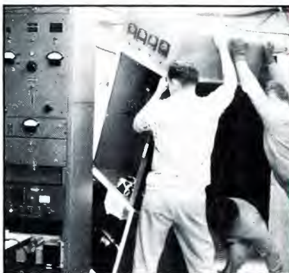
Transmitter installation work is done at KNDO-TV in preparation for station sign-on. The UHF transmitter is an RCA model, as are the frequency and modulation monitors on the left.
